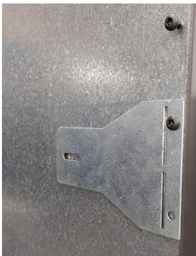
Figure 16: Nailing Flange Flat
